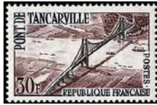
Tancarville Bridge A327
