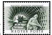
Subway Construction A225
