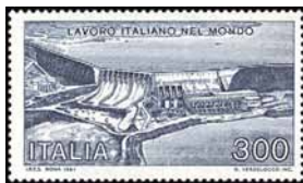
Sao Simao Dam and Power Station, Brazil — A732
