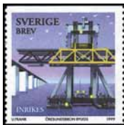
Construction of the Öresund Bridge — A708
