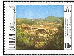
Maameltein Bridge — AP154
