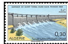
Irrigation Dam at Djorf Torba-Oued Guir — A112
