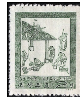
House Building — A529
