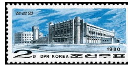
Changgwang Health Complex — A1012
