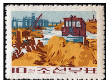
Sunhwa River Works A495
