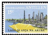
Desulphurization Plant, Lago — A102
