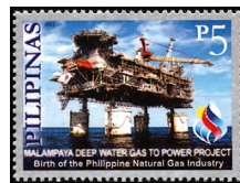
Malampaya Deep Water Gas Power Project A845
