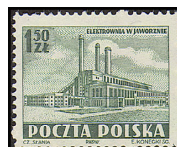
Power Plant, Jaworzno A209
