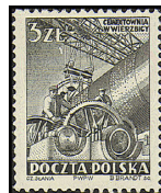
Concrete Works, Wierzbica A206
