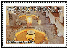
Power Station A77
