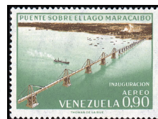
Lake Maracaibo Bridge AP56
