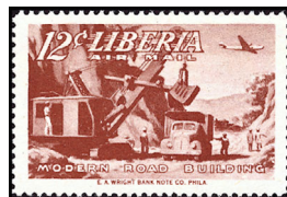
Road Building — AP22
