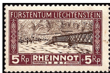
Railroad Bridge Demolished by Flood SP3
